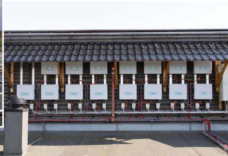
15 Delta H5A solar inverters are installed at Tveita Senter shopping center in Oslo
