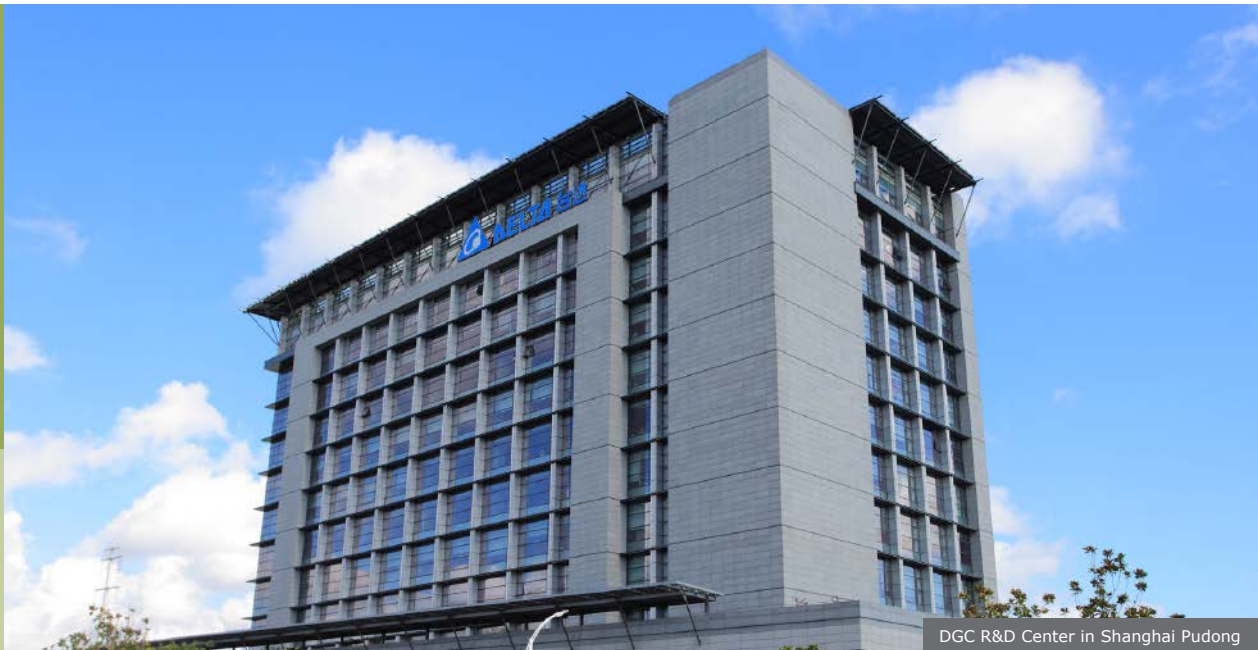
DGC R&D Center in Shanghai Pudong
