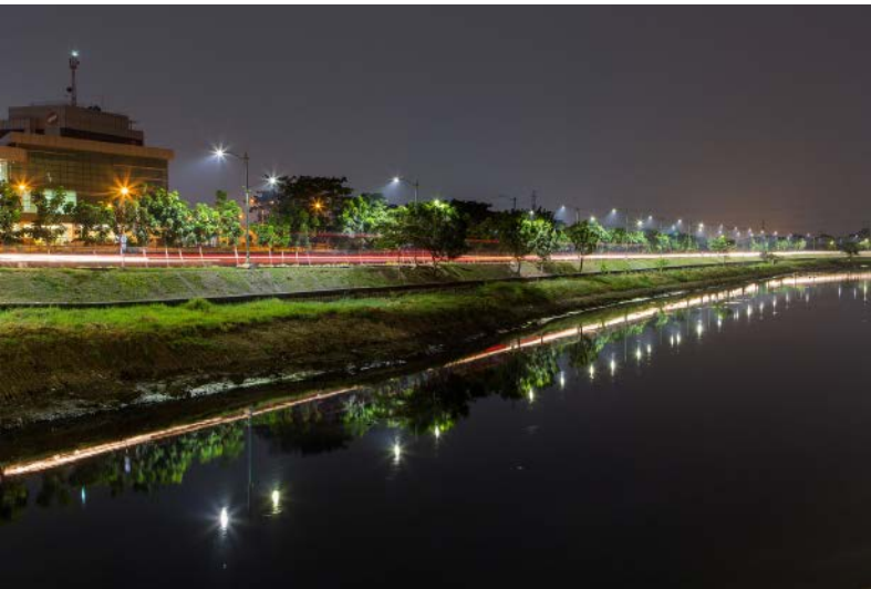
Delta's smart street lights installed on the riverside road of Banjir Kanal Timur improve safe driving
