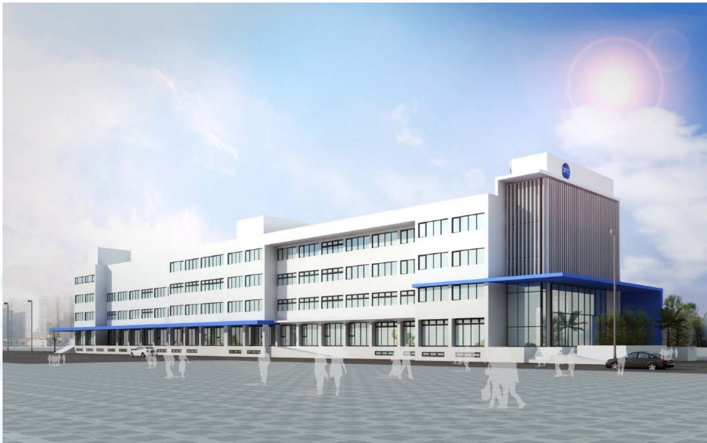
Delta's Building Automation solution creates a smart, safe, energy-efficient and comfortable office building for OPTC
